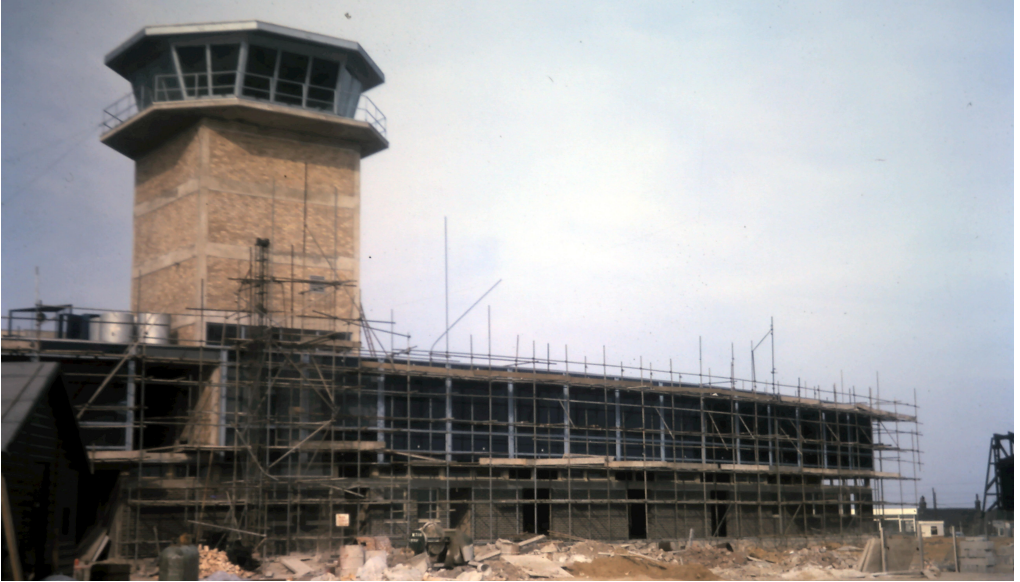
1966-67 - New Terminal construction
